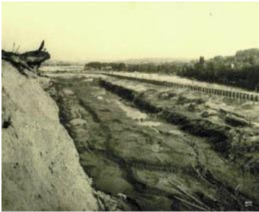
Construction of Lake Washington Ship Canal, Seattle, 1912
