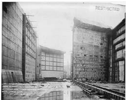
Hiram M. Chittenden Locks under construction, 1915
