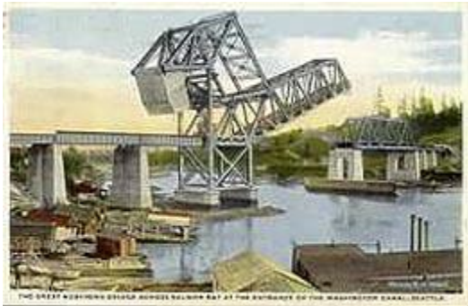
Great Northern railroad bridge (1917) across the Lake Washington Ship Canal, Ballard, Seattle
