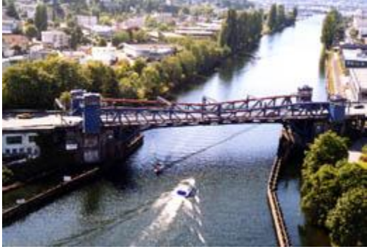
Fremont Bridge shot from Aurora Bridge, Seattle, July 2001
